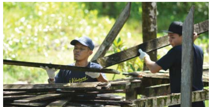
Photo: Repairing the wooden plank walkways
