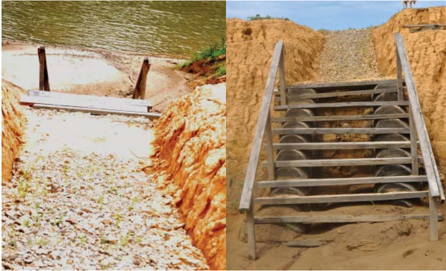
Photo: Construction of the landing stage
